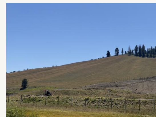
Lanes Creek Reclamation
