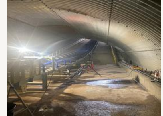
Ore loading tunnel
