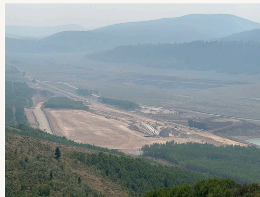
H1/NDR tipples and stockpile area
