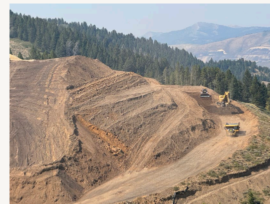
North Dry Ridge box cut
