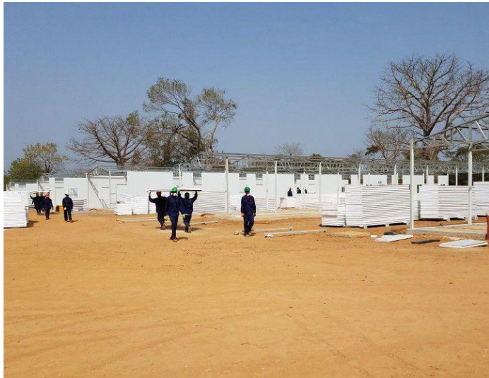
Construction of Farim Camp
